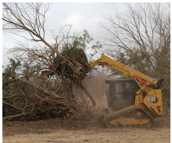
Removing invasive trees and shrubs at Fertig Prairie.
